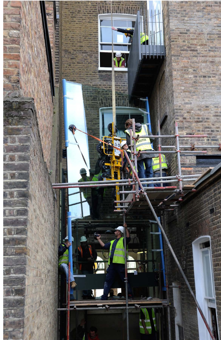
Installation of the largest double glazed unit in Europe, stretching over 2 and a half stories it
