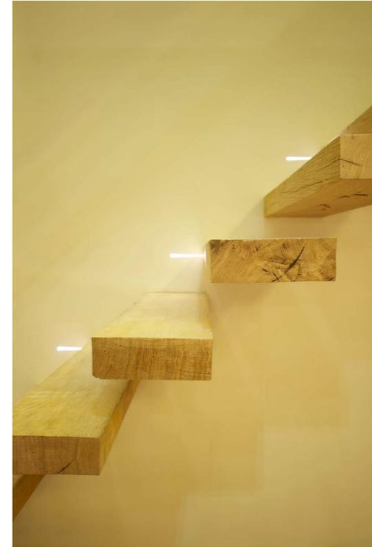
single monolithic expressed oak treads with lighting detail emphasising the single block of timber's grain and texture
