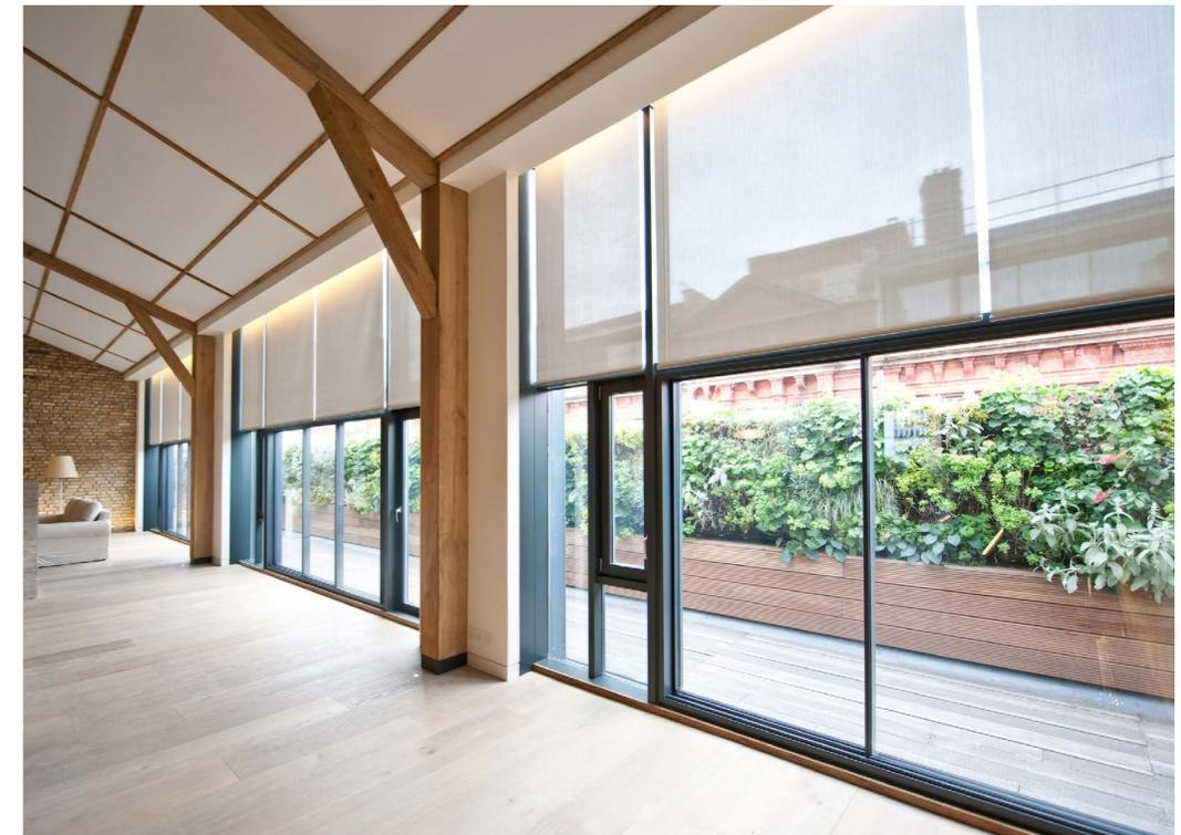
detailed ceiling lattice work, also in oak that supports an acoustic ceiling
