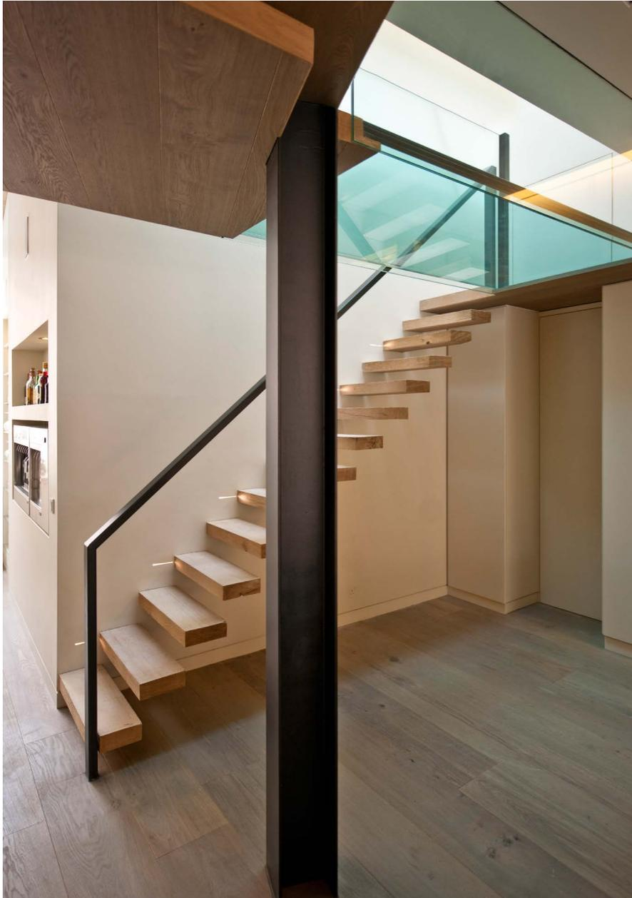
a structural glass floor connects the mezzanine level and brings light from the skylight above to both floor levels
