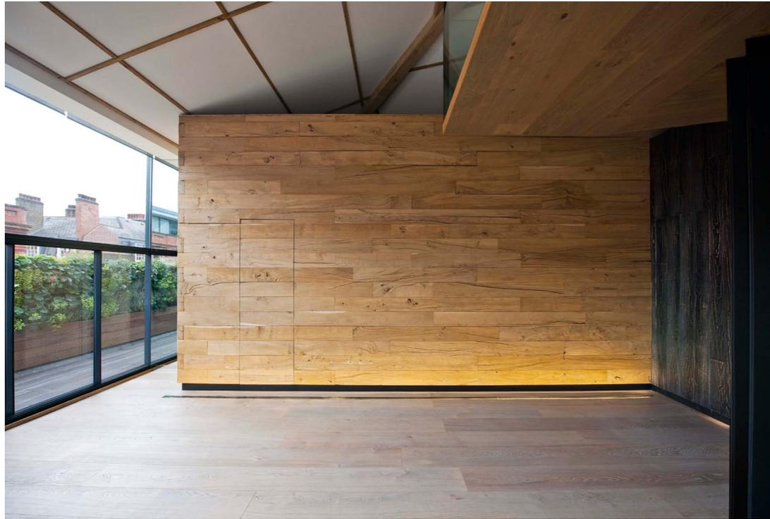
a timber boxes built out of 100mm thick, wire brushed and sand blasted oak with a caustic soda finish, with almost invisible door entries
