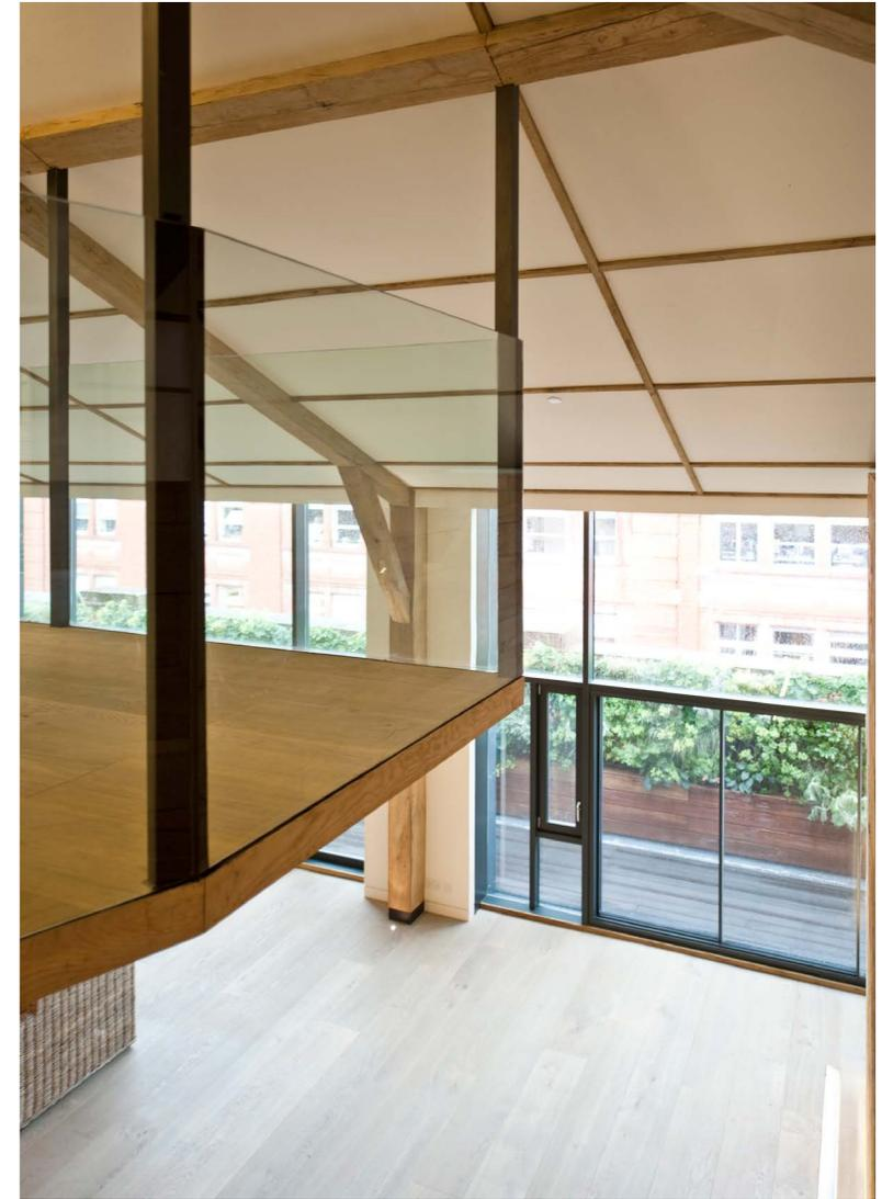
The aim was to make the mezzanine floor plate to appear floating: the structural challenge was to reduce floor thickness to the minimum possible, as a result it is only 95mm thick. This was technically achieved by suspending the floor from the steel
